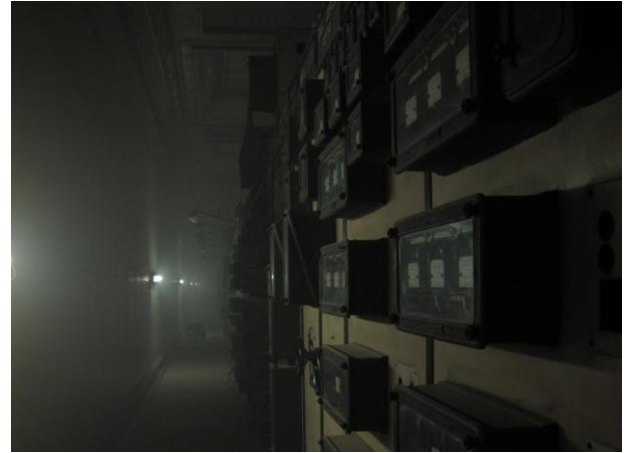
Figure 5: Machinery and marble walls in Control Room A
